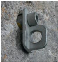
Fig. 8 Examples of self-drilling anchors (a type of expansion bolt system)
