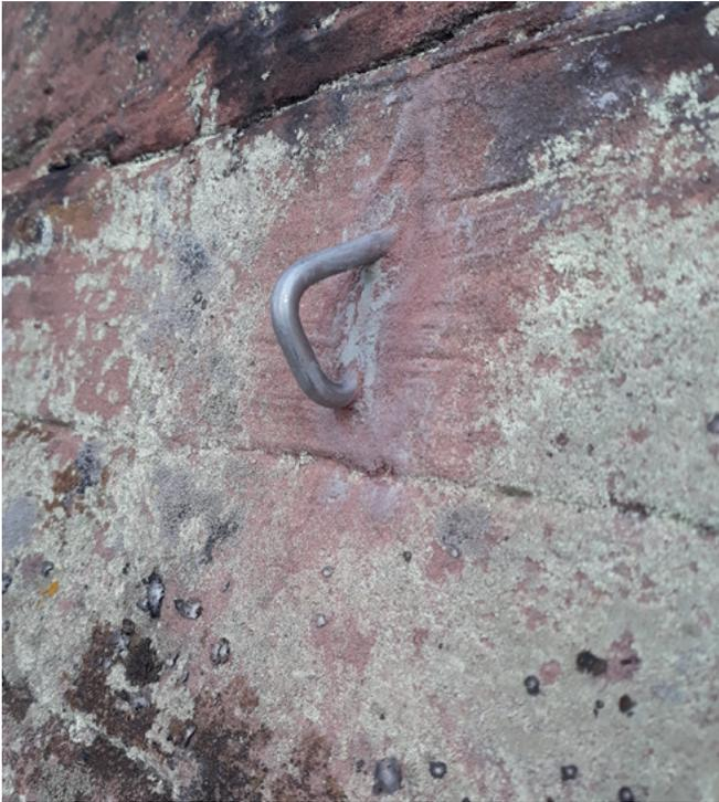
Fig. 58 Glue-in bolts in Palatinate sandstone.
