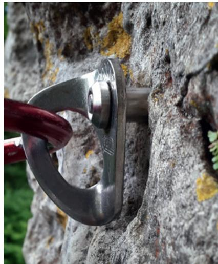
Fig. 62 This loosened drop-in anchor is evidence of the softer rock layers that are often found only a few centimeters below the rock surface in the Frankenjura. For this reason, glue-in anchors are used almost exclusively. Photo: Jürgen Kollert.
