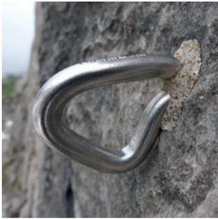
Fig. 1 Glue-in bolts can be recognized by the chemical bonding agent the „glue“ around the bolt shaft at the entrance of the borehole)
