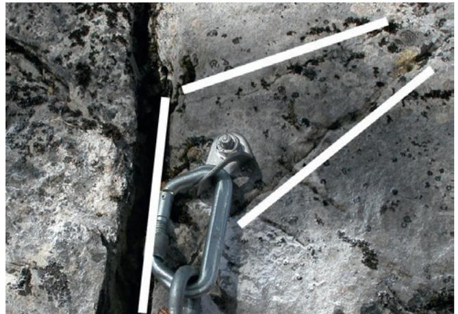
Fig. 46a This bolt was set only a few centimeters from obvious cracks and weak points in the rock.
