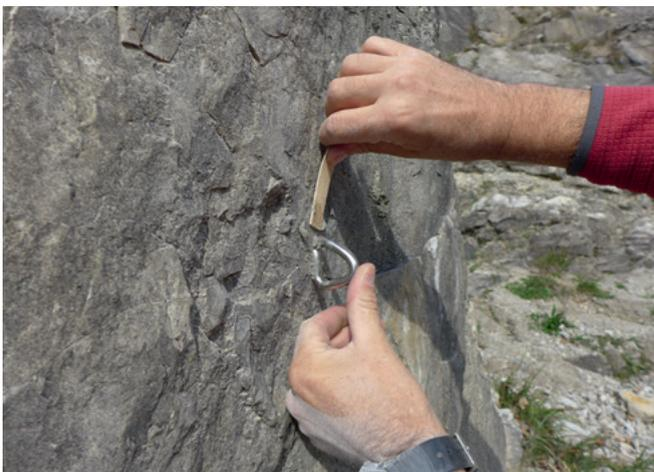
Fig. 30 The bonding agent that has leaked out from the annular gap between the bolt and the rock is smoothed out.
