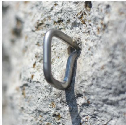
Fig. 63 Typical Böhler bolt (glue-in bolt) in the Frankenjura. Photo: Jürgen Kollert.
