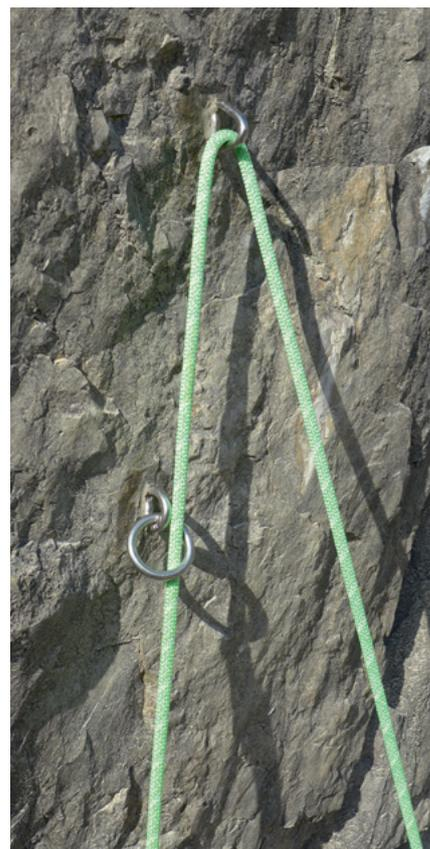
*Fig. 78c Glue-in bolts without sharp edges that can be threaded are also suitable as multi-pitch belay and rappel stations. When using express anchors, each needs to be equipped with only one chain link.*
