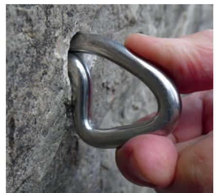
Fig. 27 Countersinking of the lower edge of the borehole with a hammer for optimal bolt placement depending on the bending radius of the glue-in bolt.
