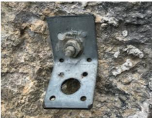
Fig. 22 8 mm wedge bolt with home-made hanger
