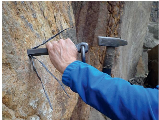
*Fig. 66 Installation of iron ring by means of lead strip*
