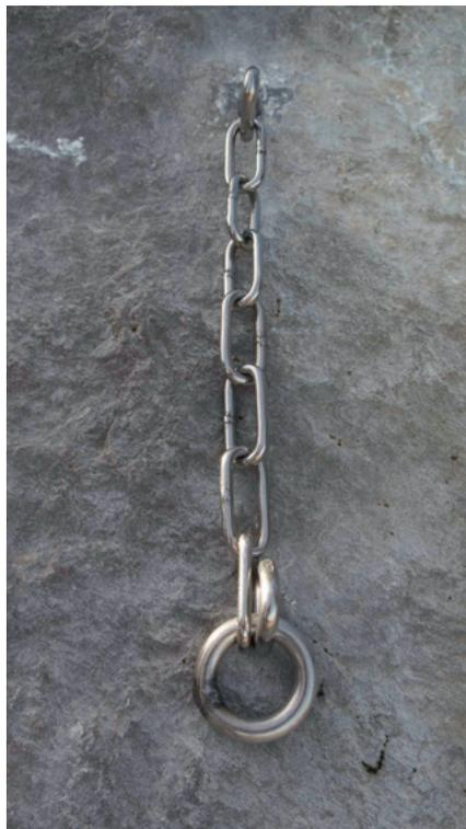
*Fig. 75 A complete system with two glue-in anchors for homogeneous, good rock quality.*
